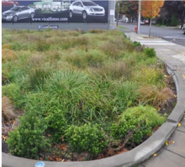
**Bioswales are critical to infiltrating urban stormwater, thereby removing water from the piped stormwater system which saves money, helps replenish groundwater, and reduces winter runoff which otherwise would erode streams and impact wetlands.**
