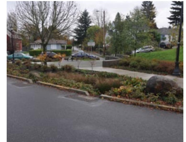
**Curb extensions, a common feature of green street designs, allow water that would otherwise be directed into storm drains to recharge groundwater where soils conditions allow for infiltration. These bioswales also calm traffic and make a more aesthetically pleasing streetscape.**
